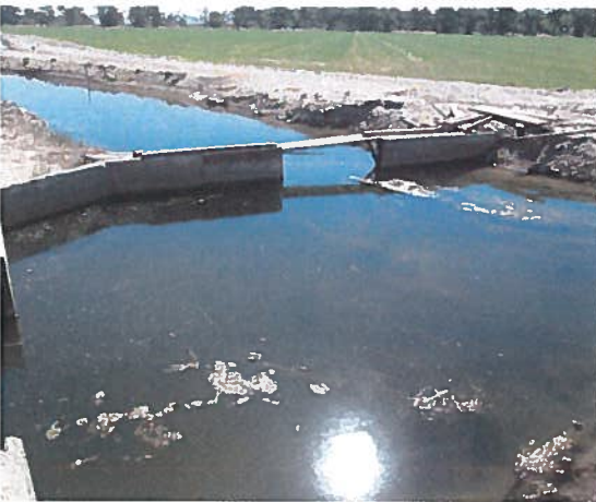
Campbell Canal Split Structure
